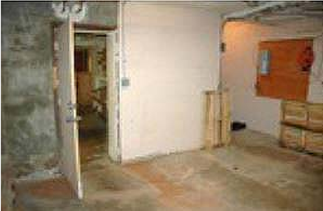
Basement storage entrance
