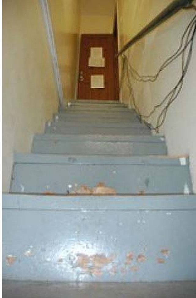
Stairs leading up from basement
