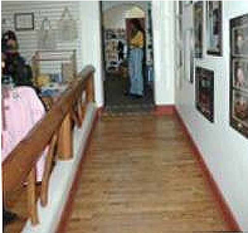
Ramp where “boot steps” have been reported
