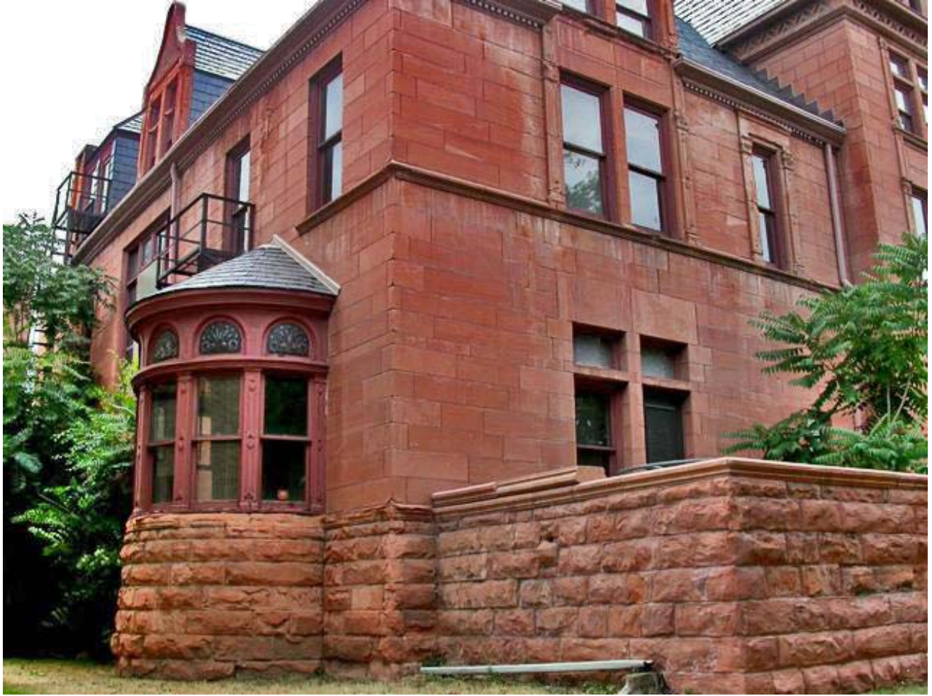
Repairs to the sandstone
