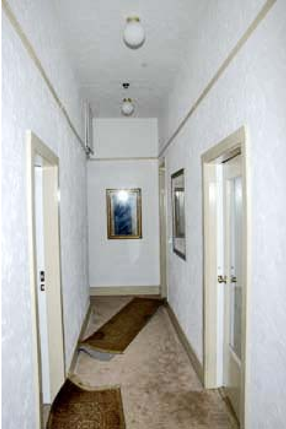
Third floor hallway
