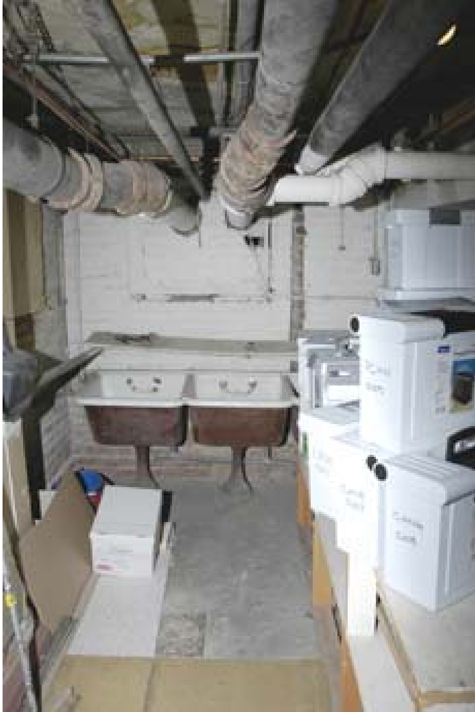
Basement Laundry room
