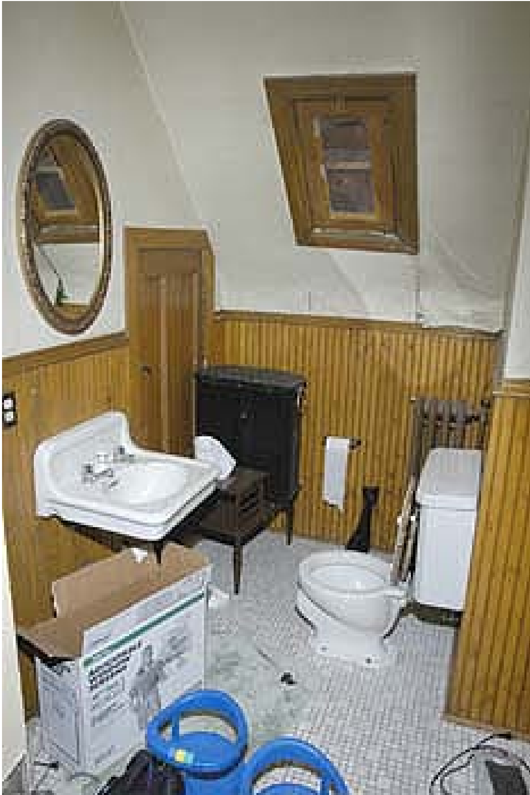
Second floor bathroom
