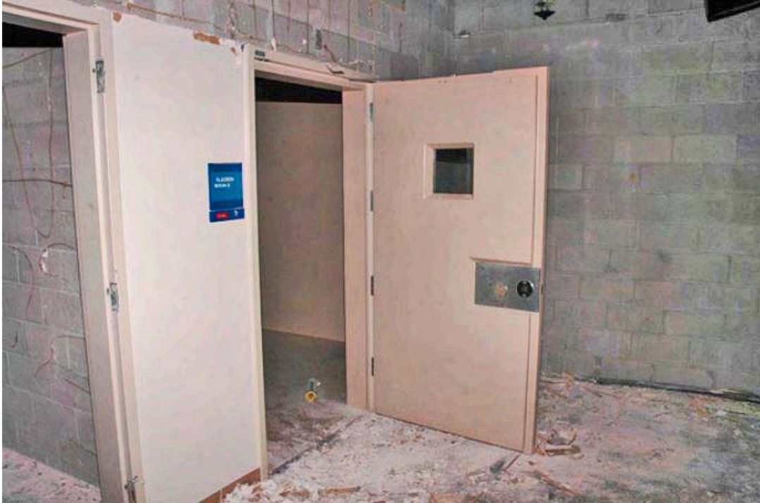
Padded room on 4 South
