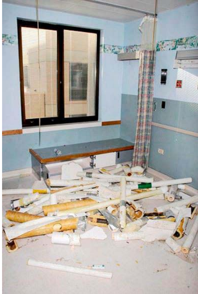
Reclamation of copper in patient room
