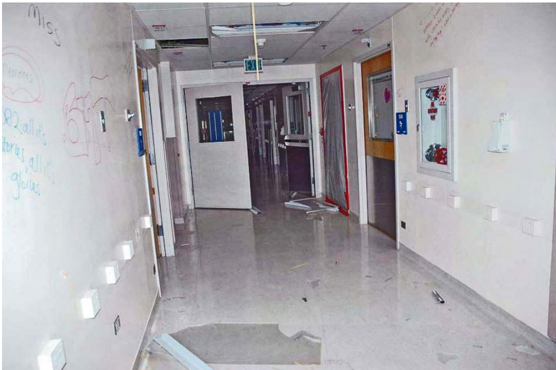
5 th Floor Hall
