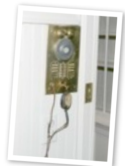
Part of the original intercom system.
